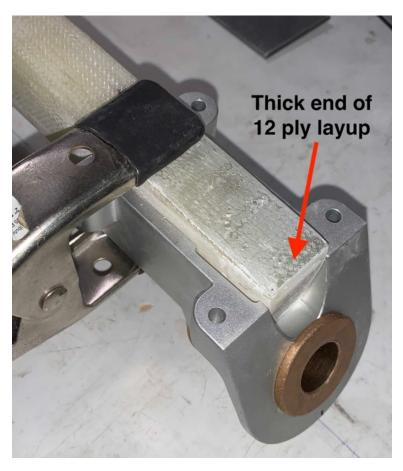
3. After cure, remove the peel ply and sand the layup so that the distance from the four lugs to the top of the NG1-L strut is even. The distance should look like this when the NG-2B is placed on the top of the strut:
